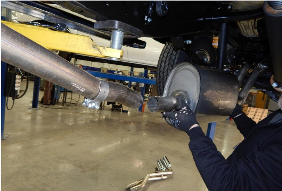
**STEP 2:** Insert the front and rear hangers into the isolators.
